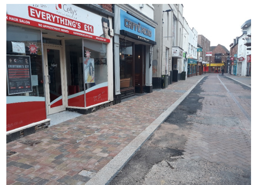
Excellent progress made along eastern footway
