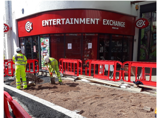
Preparing the sand bed outside City Arcade
