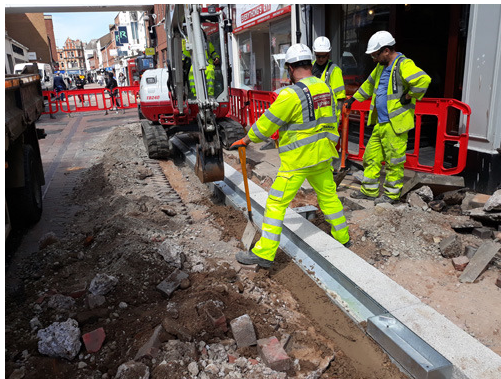
Installing new kerbs and linear drainage system outside Café Nero
